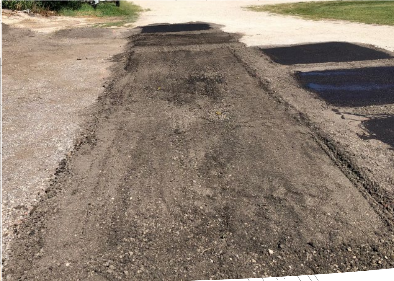
Trial Section after application of product.
